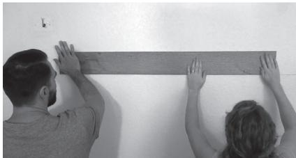
4. With the use of a pencil and a 4' level, establish a starting line across your wall at eye level. DO NOT adhere the plank until you have it placed in the right position. Once the material is adhered to the wall it will be very difficult to reposition.
