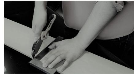
8. Planks can be cut to fit by using an electric miter saw, a hand saw and miter box or by using a square as a guide and scoring the top and bottom surface with a utility knife and snapping through the high density fiberboard core at the cut mark. If the planks are cut by hand, a sanding block will be needed to smooth the cut edges.
