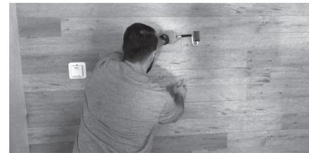
**10. Important!** To help set the Vacubond™ adhesive after the installation is complete, the wall **must** be rolled using a J-roller to insure the bond. Not using a J-roller can lead to failed adhesion. J-roller available for purchase at [www.wallplanks.com](http://www.wallplanks.com).
