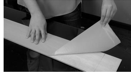
5. Starting on the left side of the room, using the starting line (and nails) as a guide, peel the paper off the Vacubond™ adhesive and position the starter row planks groove side up along your line. Press into place. If you placed positioning nails in the wall in Step 4, remove them now.
